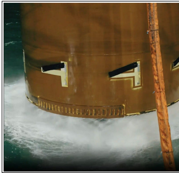
Figure 11. Jetting noise abatement technique used to install monopile foundations at Gode Wind 3 in Germany (Ørsted, 2024)
