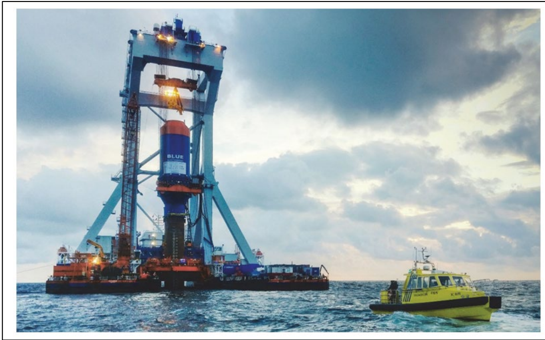
Figure 10. Fistuca's BLUE Hammer deployed on an installation vessel placed on top of a monopile (NatureScot, 2019)
